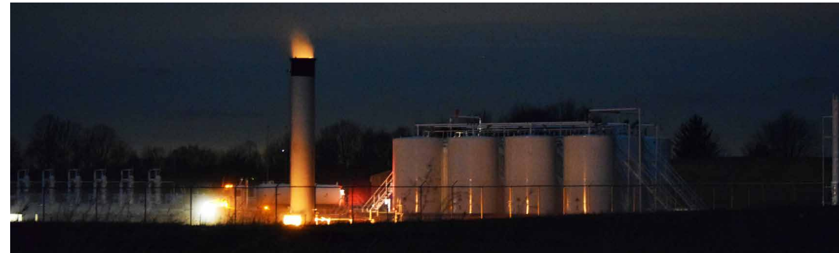
Green completion stack on a fracking well pad in Carroll County, Ohio. Photo by Ted Auch, 2015. These photos and more can be found in our online albums: fractracker.org/photos
